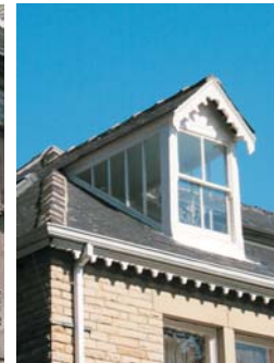
(k) Dormers are characteristic of some Victorian properties. Note the glazed cheeks.
