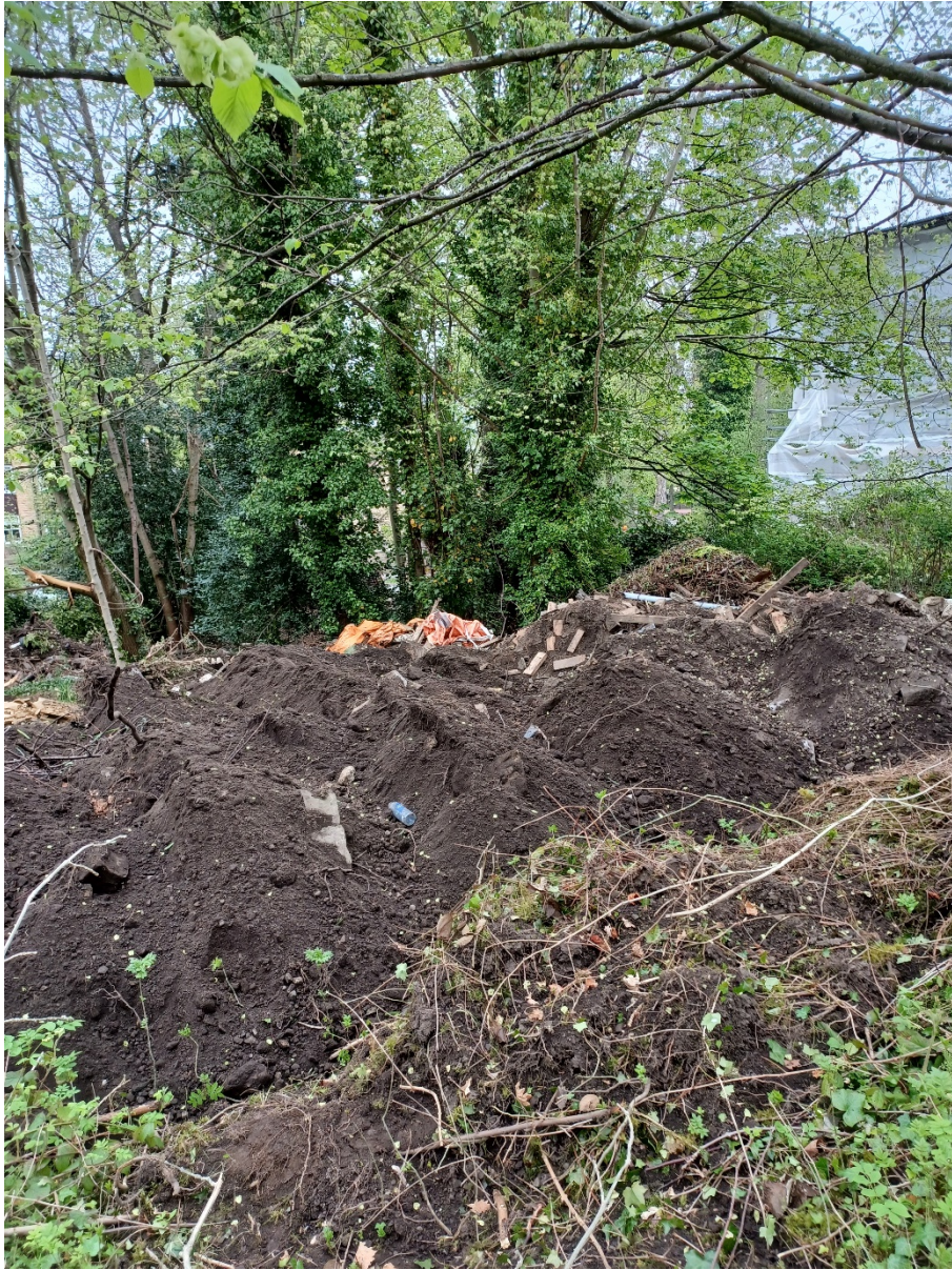
Image 3. Level changes in the rooting area of protected trees, caused by heaping of construction spoil within the woodland.
