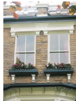
(i) Sliding sash windows constructed in timber.
